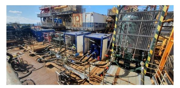
After the first sample was taken, the fluids were deemed of a quality that could bypass the RFV4000 Absorbent media units and increase the flow rate up to the maximum pumping rate of 260 m $^3$ /hr and overboard directly from the Hi-Flow $^{TM}$  oil in water coalescers.
